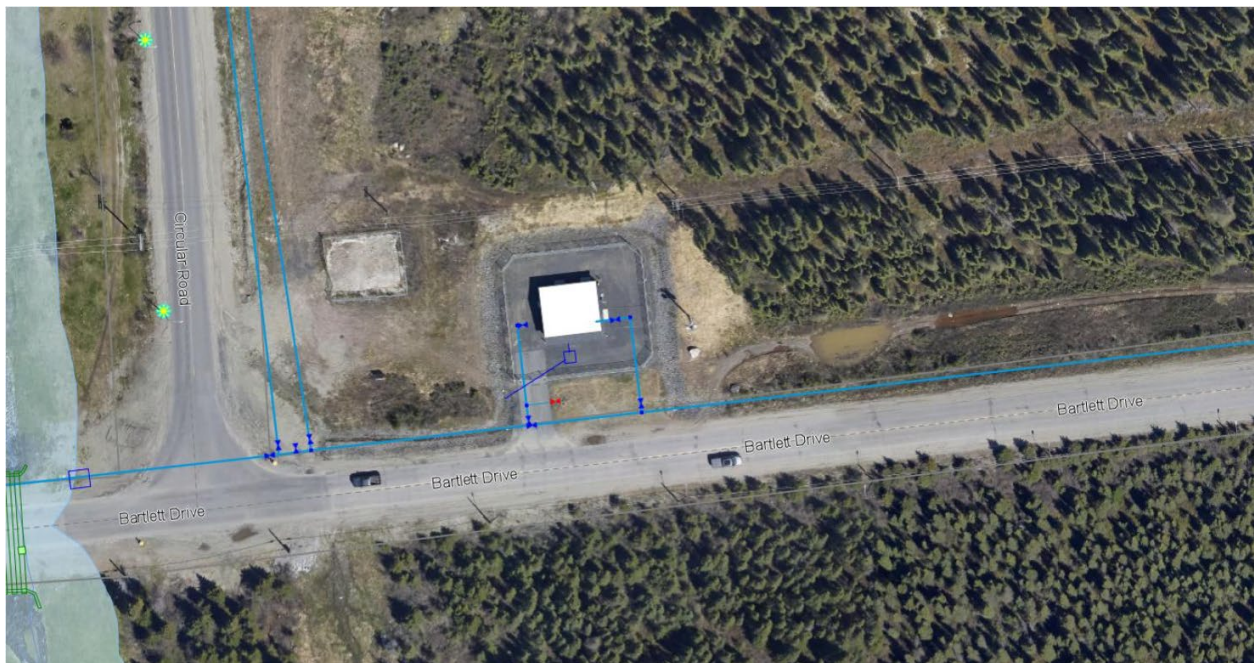
Figure 1 250Ø ductile iron water main leading to Bartlett booster station.
