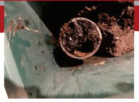
4 Inch Sewer Pipe 80% Blocked Results From Blocked Sewer Lines
