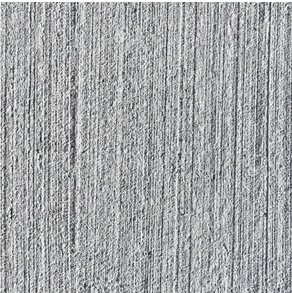
Concrete Sidewalk - broom finish and saw cut
